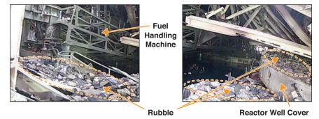
FIGURE 2.6 Views of the damage on the refueling deck in Unit 1. Note: See http://www.tepco.co.jp/nu/fukushima-np/roadmap/images/d141225\_10-j.pdf for more images. SOURCE: Tateiwa (2015).
