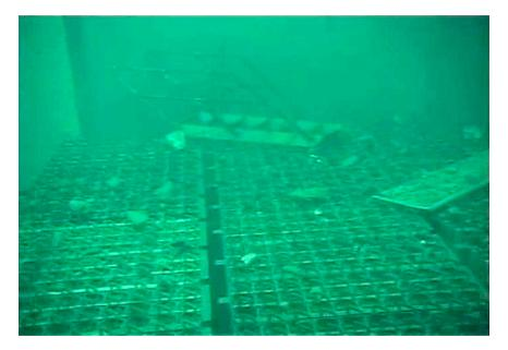
FIGURE 2.11 Debris on top of fuel racks in Unit 4 pool. SOURCE: TEPCO (2012a, Attachment 9-5, Figure 7).
