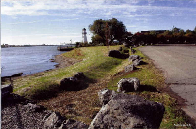
Before-and-after photos showing soft engineering techniques at DTE's River Rouge Power Plant, Nativescape
